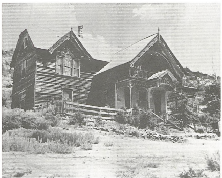
FIGURE 2-13. Stoddard House (Block 5, Lot 9). A unique detailed home in comparison with others in the community.
